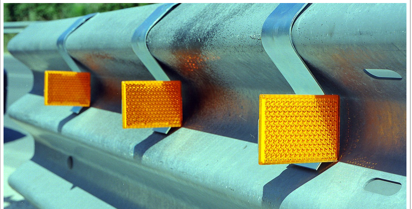
Catadiotri su guardrail / Reflectors on a guardrail
